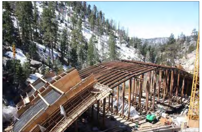
Flatiron Construction of Big Bear bridge construction
