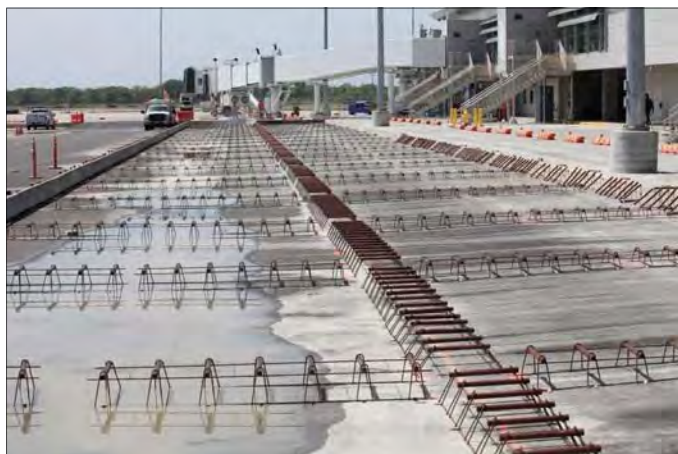
Flatiron Construction concrete apron for Terminal 2 at San Diego International Airport
