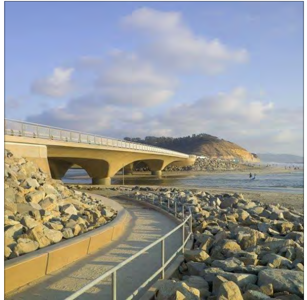
Flatiron Construction of the completed N. Torrey Pines Dr. bridge just before entering Del Mar
