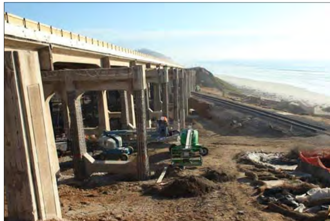
Flatiron Construction retrofit for Torrey Pines Bridge
